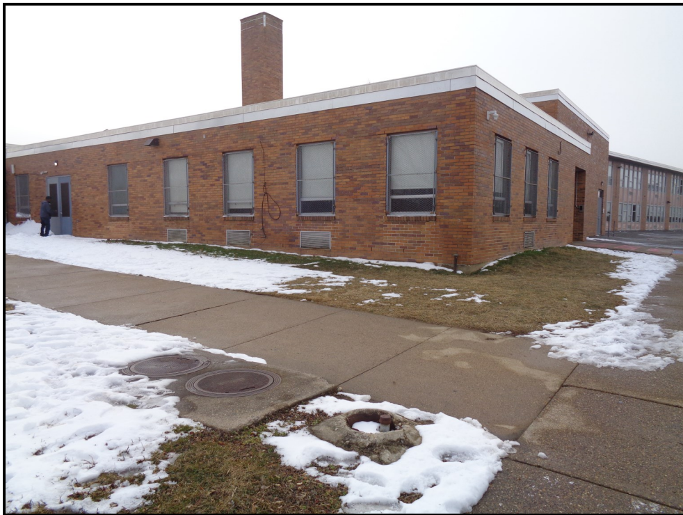
Photograph 9: View of a UST fill and vent pipe located at the northern corner of the elementary school building.
