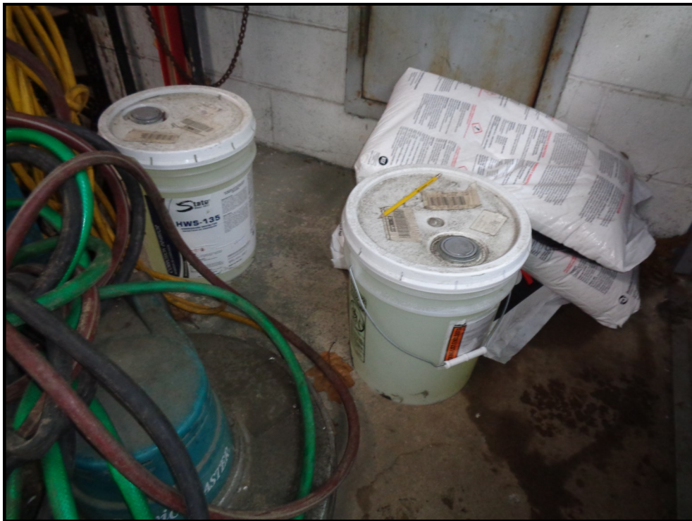
Photograph 17: View of two (2) 5-gallon buckets of corrosion inhibitor used for hot water heaters were located within the maintenance area/boiler room of the elementary school.
