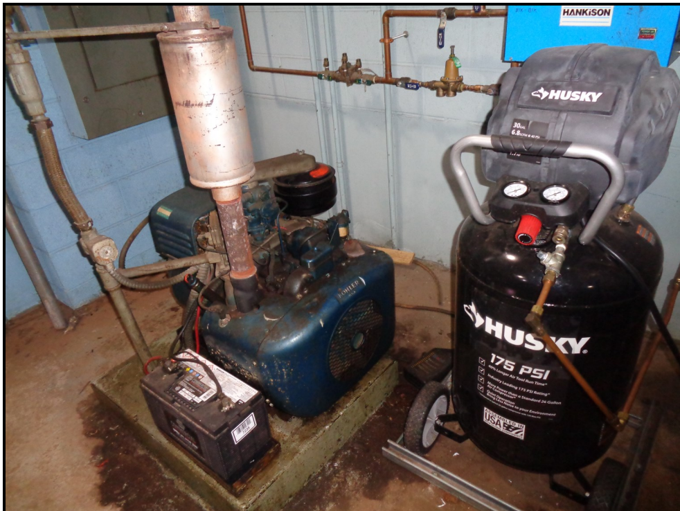
Photograph 13: View of a compressor and a lead acid batter located within maintenance area/boiler room of the elementary school.
