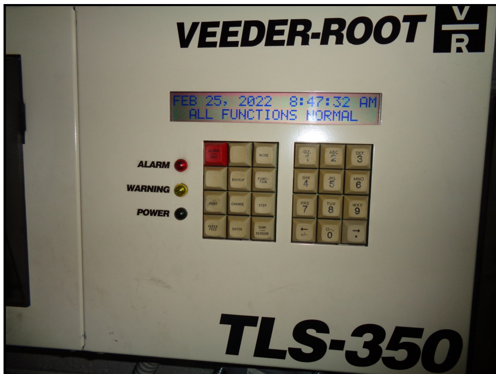
Photograph 29: View of a Veeder-Root system associated with the diesel UST located on the subject property.
