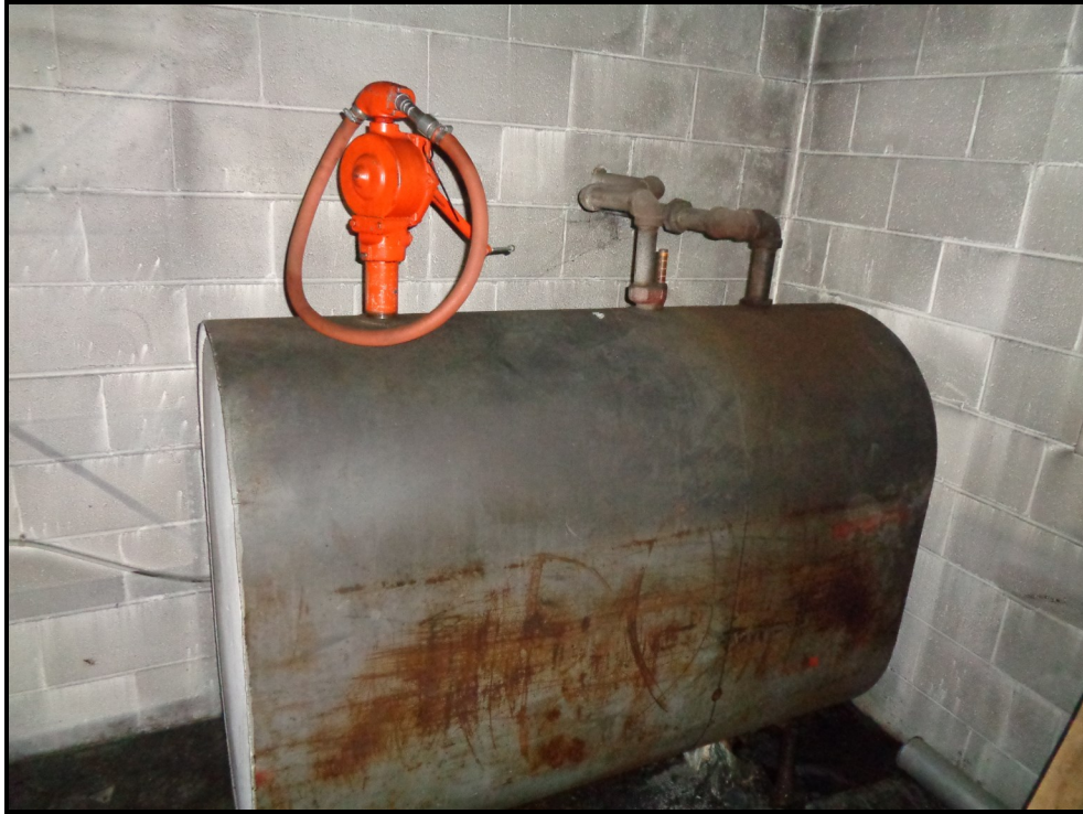
Photograph 26: View of a 275-gallon heating oil tank within the school bus garage.
