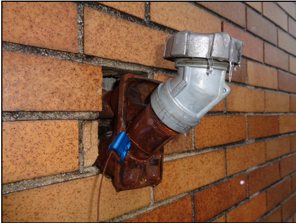
Photograph 28: View a fill and vent port associated with the 275-gallon AST on the outside of the school bus garage.
