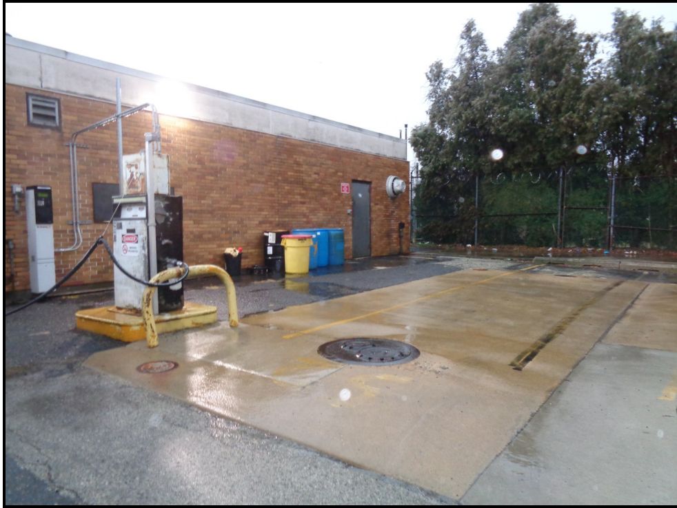
Photograph 18: View of a diesel and gasoline pump (gasoline disconnected) and diesel UST location associated with the school bus operations on the subject property.
