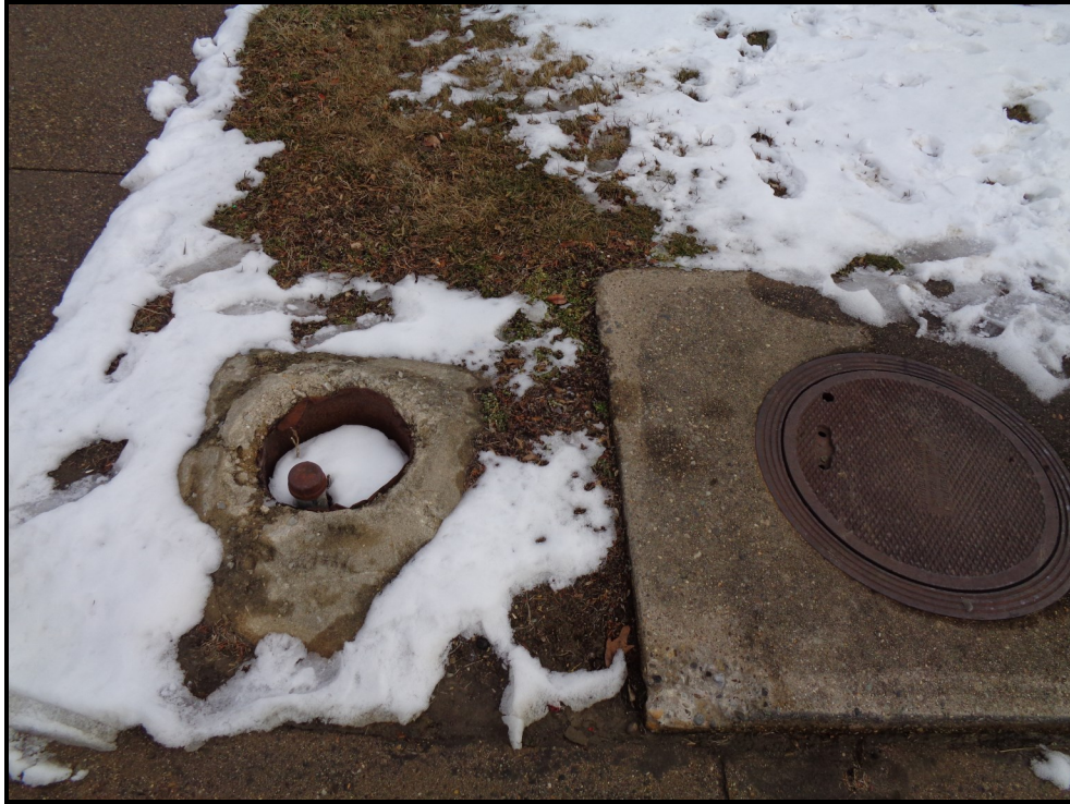
Photograph 8: View of a UST fill pipe located at the northern corner of the elementary school building.
