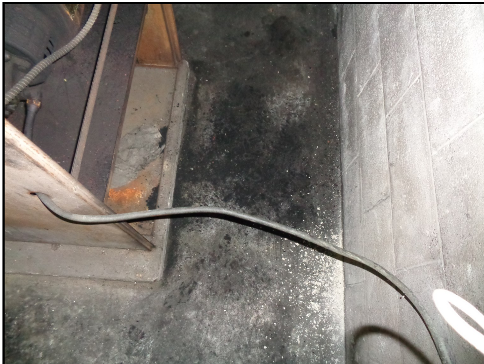
Photograph 31: View of staining behind a heater located within the school bus garage.
