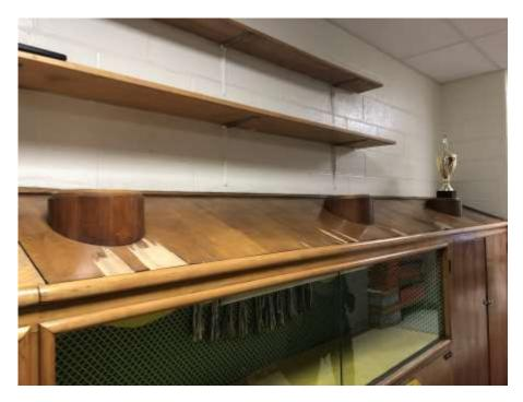
Photograph 6: Evidence of water damage on top of cubbies in the hallways.
