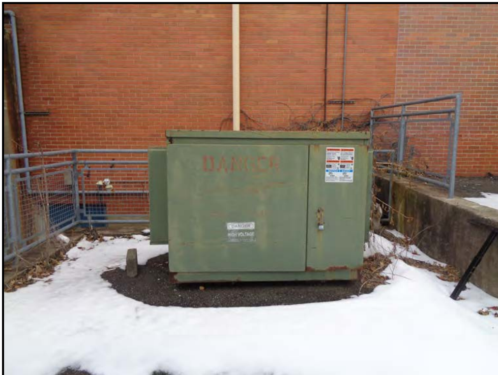
Photograph 13: One (1) pad-mounted transformer was observed to the north of the building on the subject property.
