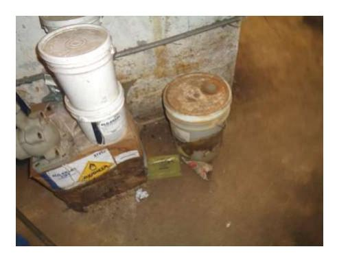
Photograph 7: Carboard box with visible mold growth.
