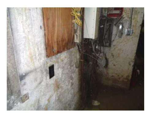
Photograph 5: Wood wall mount with visible mold growth.
