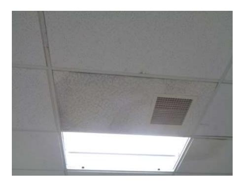
Photograph 3: Examples of stained ceiling tiles observed throughout.
