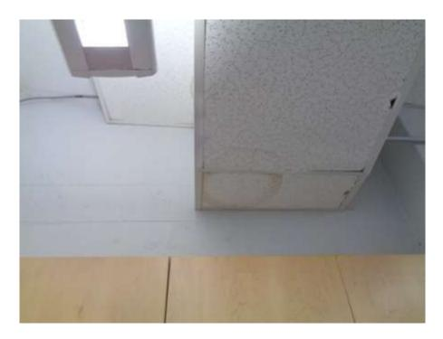
Photograph 4: Examples of stained ceiling tiles observed throughout.
