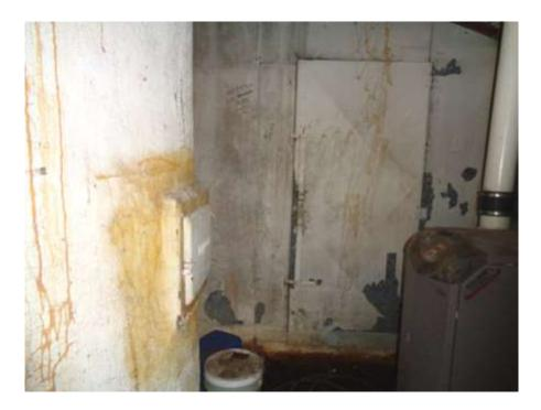
Photograph 6: Air handler unit with visible mold growth.
