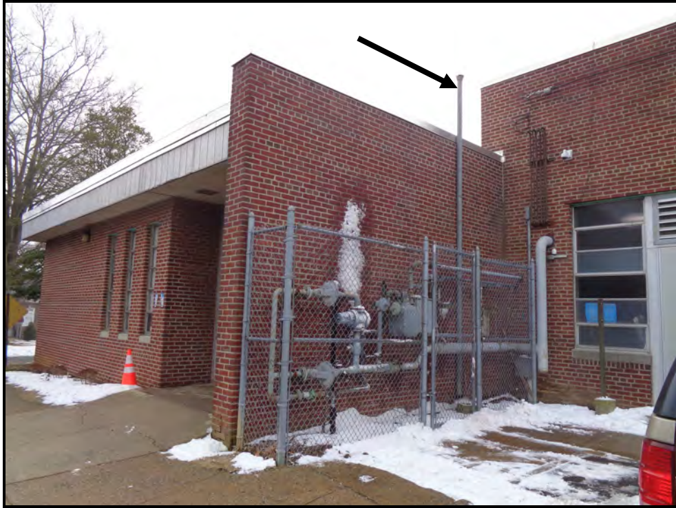
Photograph 5: View of the UST vent pipe, located on the north side of the school.
