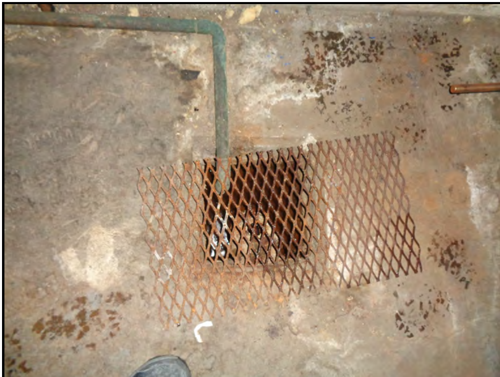
Photograph 8: One (1) floor drain with water pipe being discharged, located in the boiler room of the school's basement.
