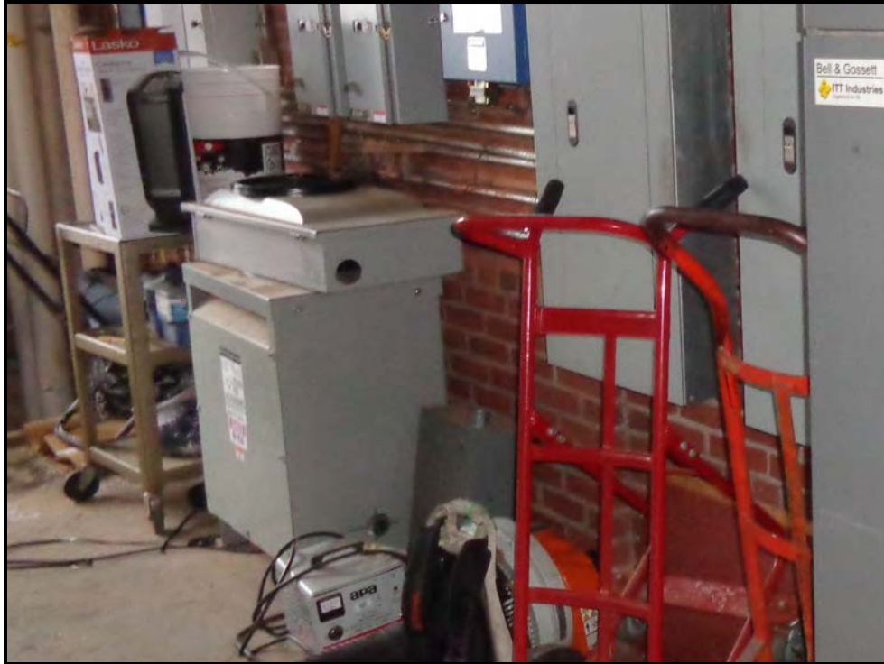
Photograph 7: One (1) transformer observed in the boiler room of the school's basement.
