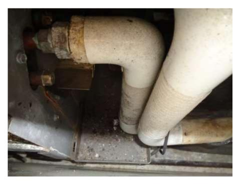
Photograph 8: Fiberglass insulation located inside classroom unit ventilator in Room 105.
