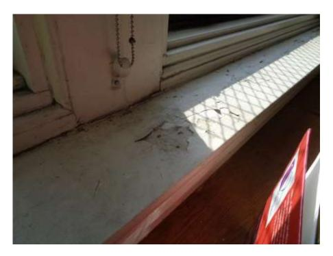
Photograph 5: Typical windowsill damage in Room 105.
