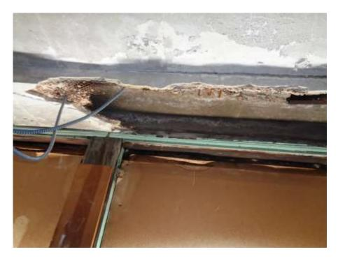
Photograph 7: Damaged plaster and exposed wood window framing in Room 105.
