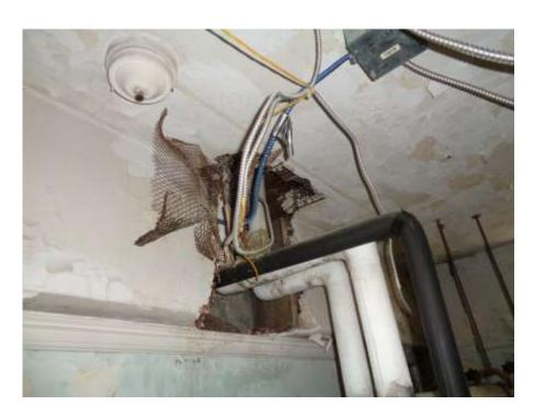
Photograph 9: Damaged plaster, fiberglass pipe insulation and exposed wood window framing in Room 209
