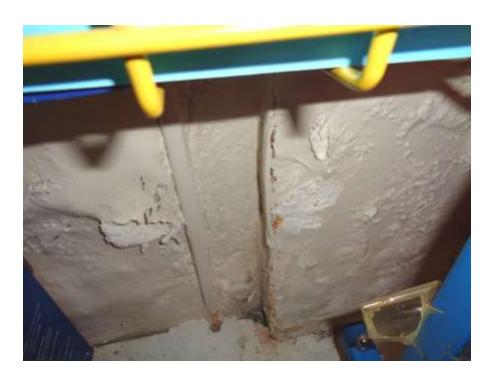
Photograph 1: Significant water intrusion on Plaster walls in Room 009.
