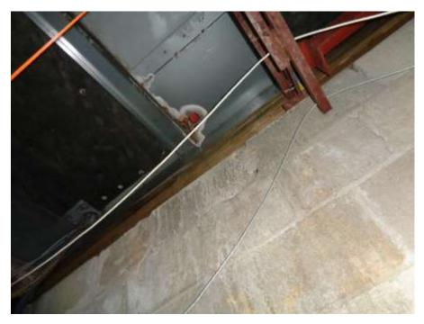
Photograph 4: Potential leaking point above ceiling tiles near main office.
