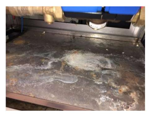
Photograph 11: Previous water building in Classroom Unit Ventilator.
